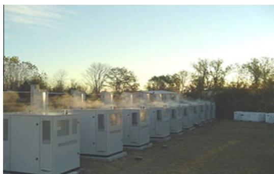
**Fig. 12.** GenSys® fuel cell system as off-grid distributed generation [271].
